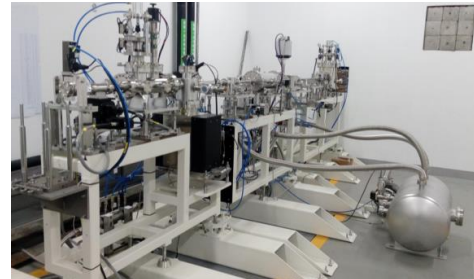
Fig.6 Installation is complete
