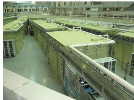
Hutch construction site
